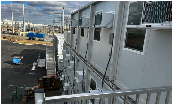
FLEX units for data center project in Mid-Atlantic
