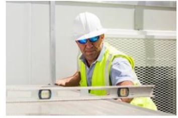
At the job site
