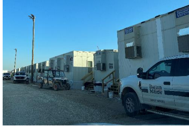
Modular trailer and complexes line up on a 2.3-square-mile battery manufacturing campus to bring a leading automobile manufacturer closer to their EV production target.
