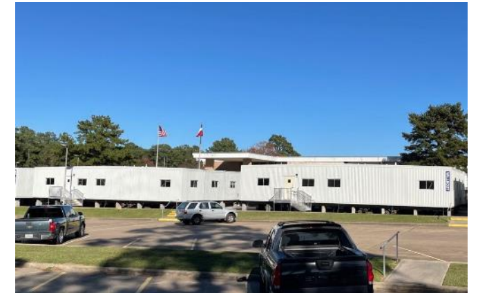
WillScot Mobile Mini delivered and installed 16 modular floors, fully furnished in 2 weeks to support a new construction project in Conroe, Texas
