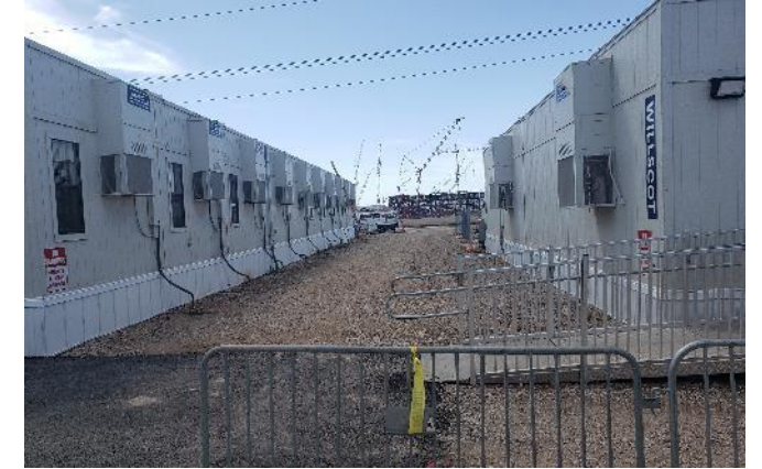
WillScot Mobile Mini set up several mobile offices and storage containers on a semiconductor manufacturing site to be used over the next 2 years.
