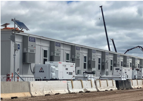
Modular complexes reinforce a data center mega project in Wisconsin
