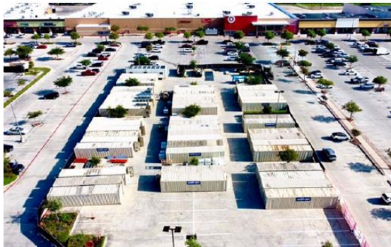
Storage containers, mobile offices, fencing, dumpsters and port-a-johns used for a Target remodel in Brownsville, TX.
