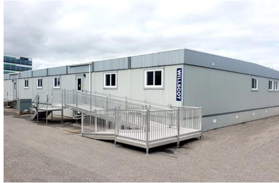
An 8-unit complex used for additional screening space for Anna Leberge Hospital located in Montreal. The entire project was ordered and fulfilled in one month.
