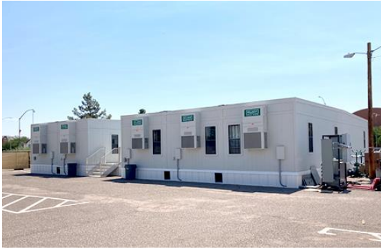
McCarthy using modular complexes during a 24-month project to construct a new Applied Research Building at the University of Arizona.
