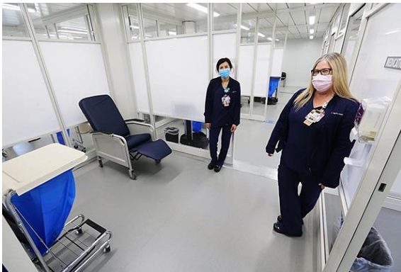
Memorial Hospital in Bakersfield upgraded from a tent to 16 FLEX floors to be used as COVID-19 examination and treatment rooms.
