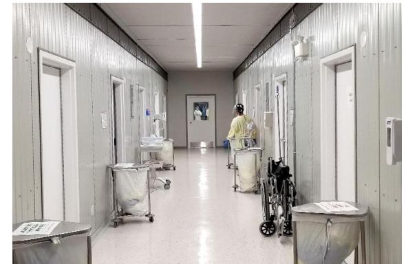
The Jewish General Hospital in Montreal, QC, is using 14 modular buildings for overflow testing and staffing space.
